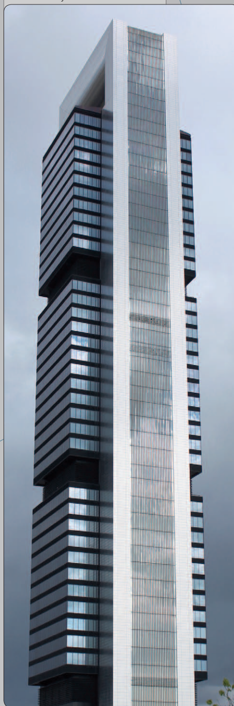
Madrid - Caja Tower
