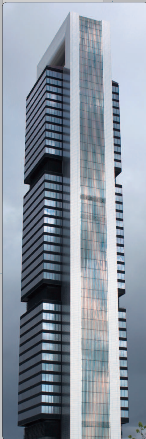
Madrid - Caja Tower
