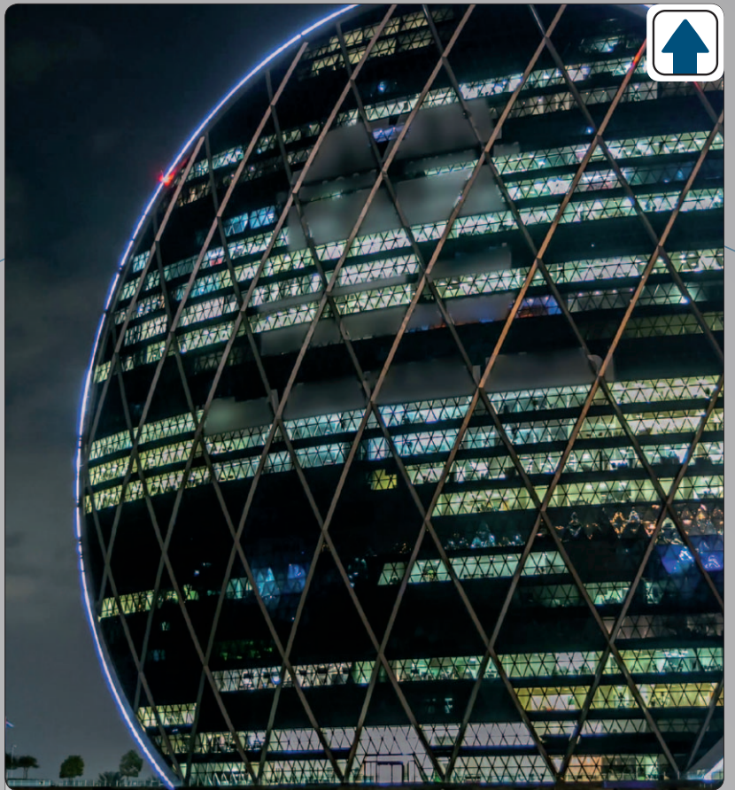
Abu Dhabi - Aldar Headquarters
