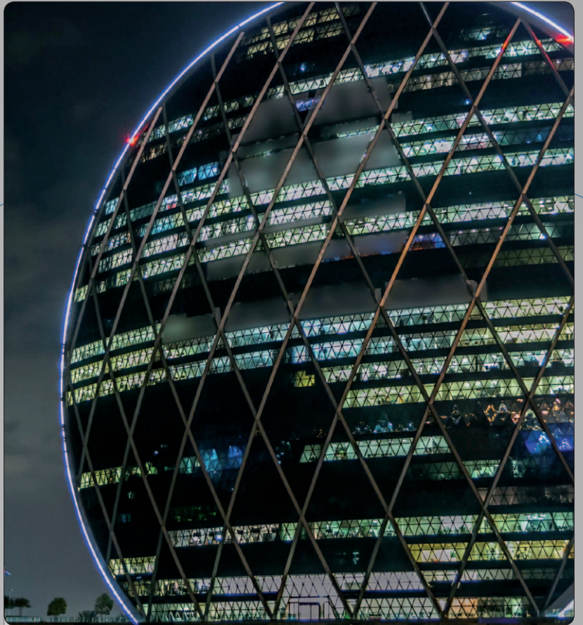
Abu Dhabi - Aldar Headquarters
