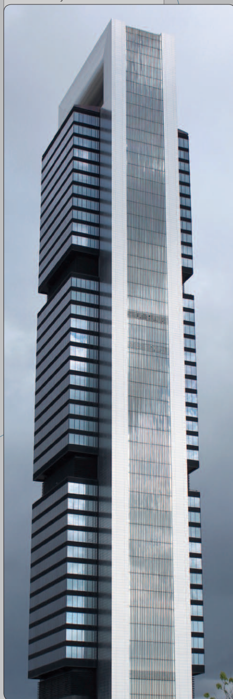
Madrid - Caja Tower
