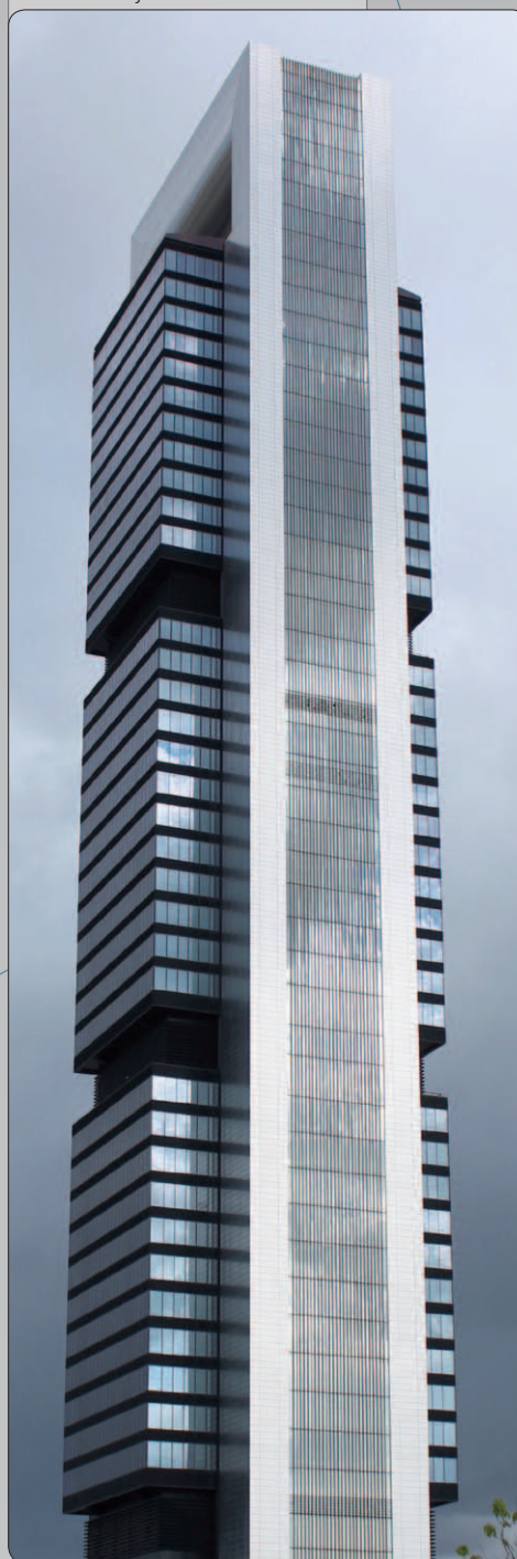
Madrid - Caja Tower
